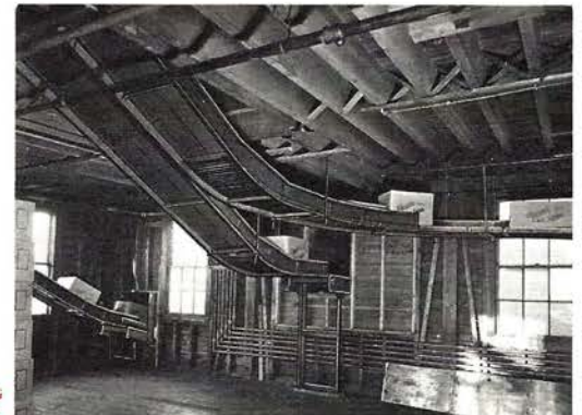
ABOVE: Small cartons of candy bars are lowered by Slides from overhead Belt Conveyors to convenient working height for packers. The slide beds are a combination of sheet metal and small close spaced rolls. The cartons are packed in large shipping cases on Roller Conveyor line in foreground and dispatched to sealing and shipping.
