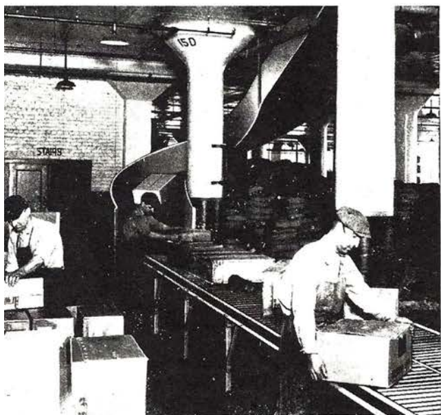
ABOVE: In a large Chicago warehouse, cartons of electrical supplies are lowered by Steel Slide to Gravity line in shipping room. Lower end of line is curved to discharge in desired direction. Installed around column to conserve floor space.
