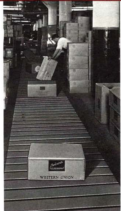
ABOVE: Slat Conveyor used for taking stock from warehouse to shipping room. Handles cases and cartons of all sizes which are loaded directly onto conveyor at any point along the line. The conveyor is installed flush with floor and can be walked on or trucked over, while in motion, without interruption to traffic.
