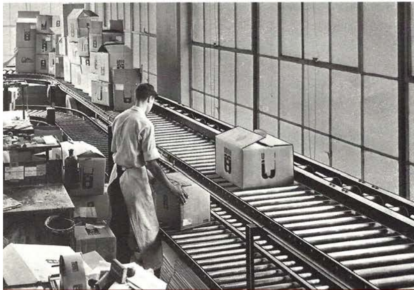
BELOW: Start of double deck conveyor in view at right showing construction of lower deck. The upper deck carries packages for parcel post and lower deck for express.
